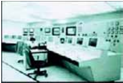
Internet remote monitoring and control.
